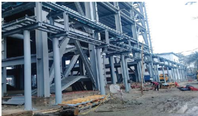
ACI Limited (Utility Bridge BBT-1 & 2), Naryangonj (1245 Rft)
