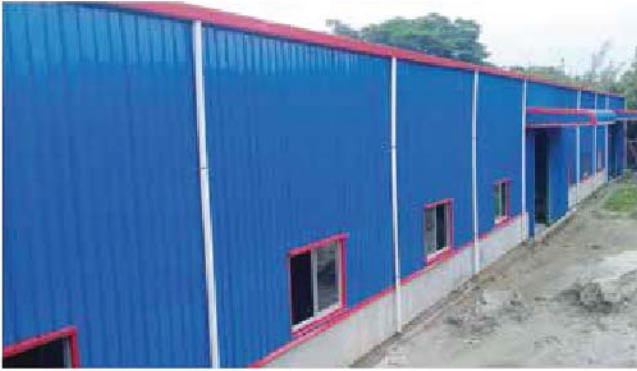
NJC Ceramic Bangladesh Limited, Workshop Building, Dhamrai, Dhaka (14270 Sft)
