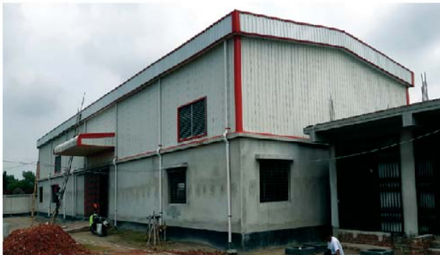
Moho Plastic Factory, Meril Road, Pabna (5632 Sft)
