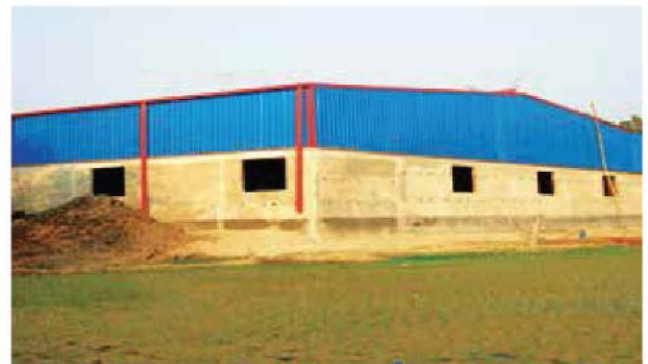
Padma Tank, Rajendropur, Gazipur. (10000 Sft)
